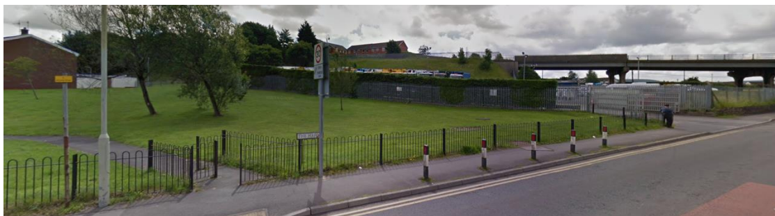
Image 4– Photograph of the site (looking SE) with the A465 running at high level in the background prior to works
