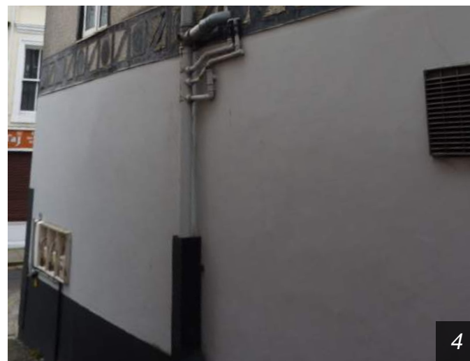
4. Pipes with protective cover, meter boxes and vent along side street.
