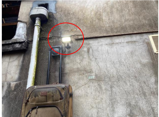
Photo 12: Security Light at the Rear (Circled)
