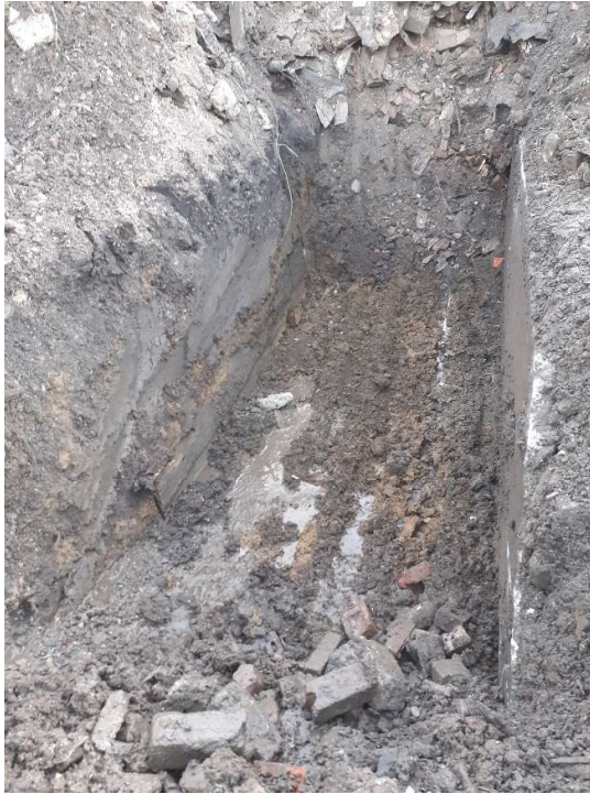
Plate 35: Excavation through Stockpile 10B to underlying natural clay.
