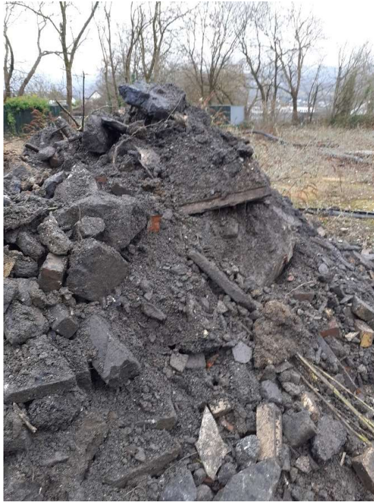
Plate 7: Stockpile 1C overview showing the varied composition and size of demolition material.
