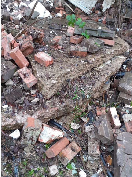
Plate 13: Fragments of reinforced concrete slabs and whole bricks of Stockpile 4.
