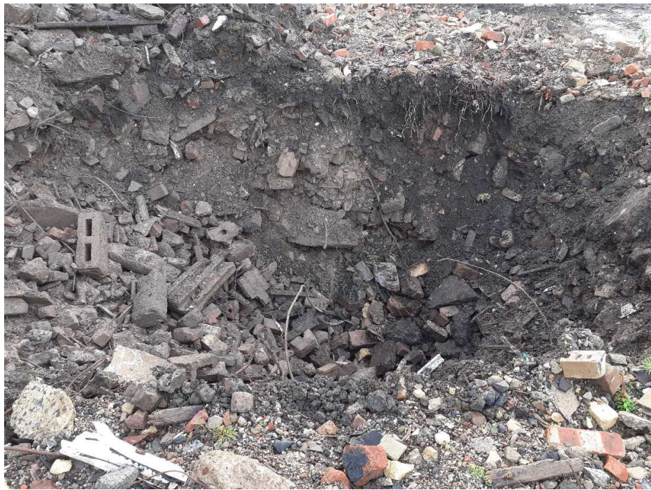
Plate 30: Excavation into Stockpile 9A with fragments of concrete, concrete blocks, brick, pipes, rebar wood and other demolition material.
