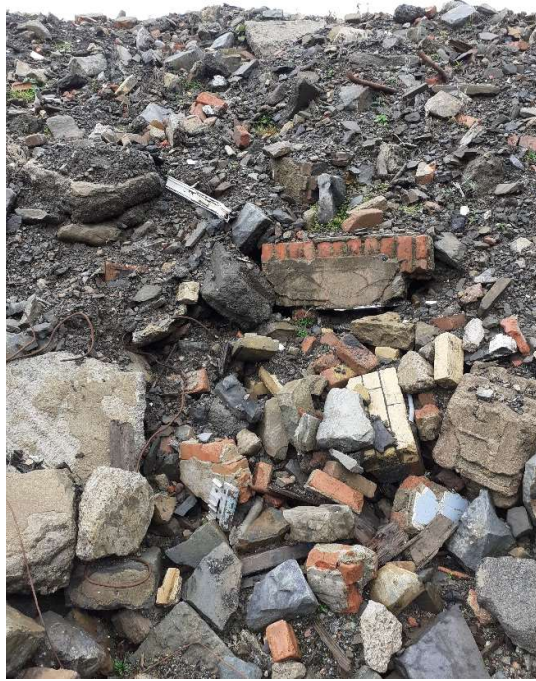
Plate 19: Overview of coarse gravel to boulder-sized demolition debris in Stockpile 6C.
