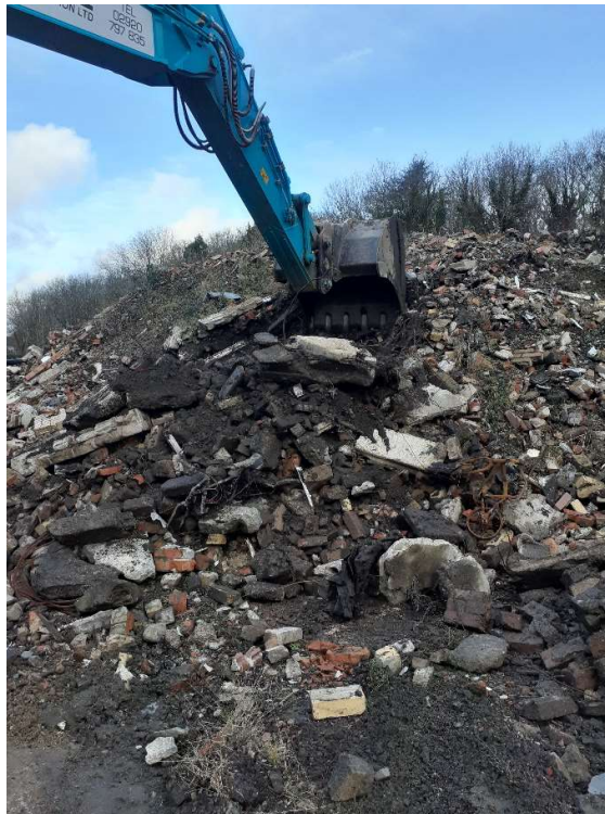
Plate 36: Overview of Stockpile 10C.
