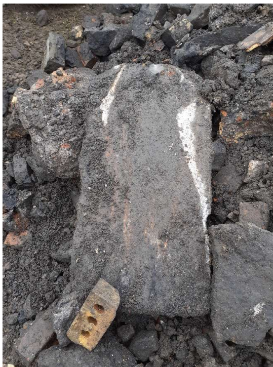
Plate 4: Fragment of concrete slab removed from Stockpile 1.
