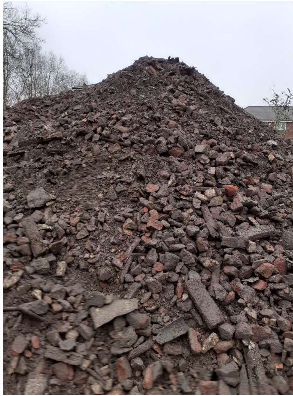
Plate 9: Overview of stockpile 2C showing possibly processed demolition materials.
