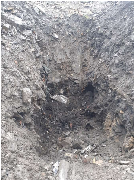
Plate 26: Pit excavated into Stockpile 7C.
