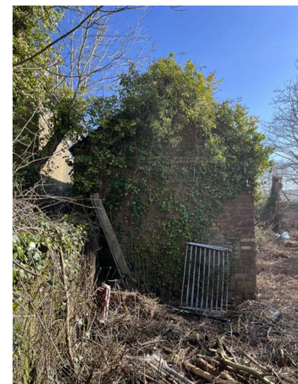
P9 Southwest elevation view
