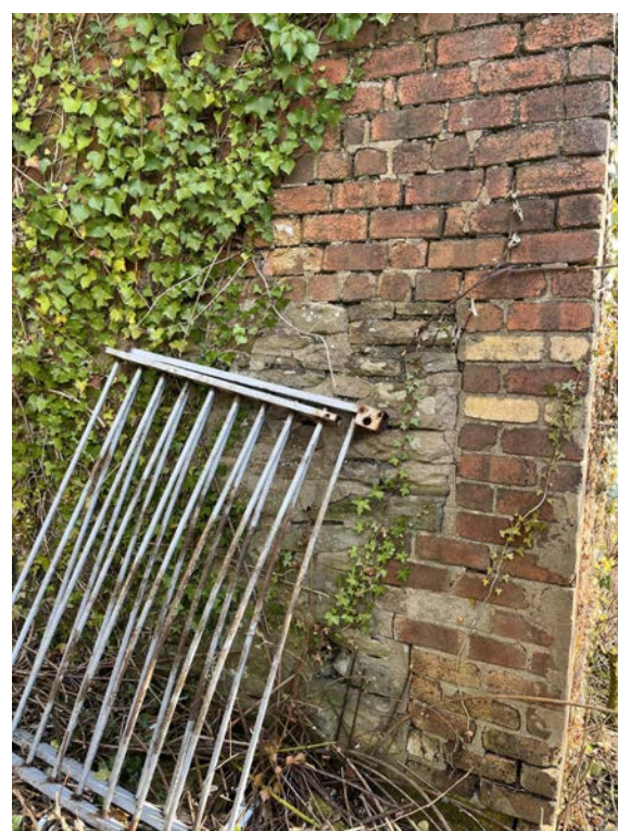
P10 South corner showing the different wall materials.
