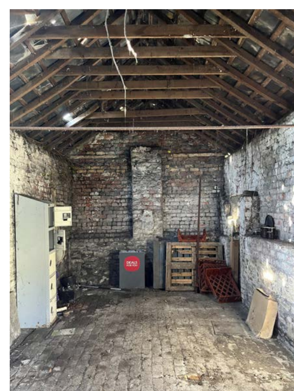
P16 internal view facing west showing the space and roof trusses.
