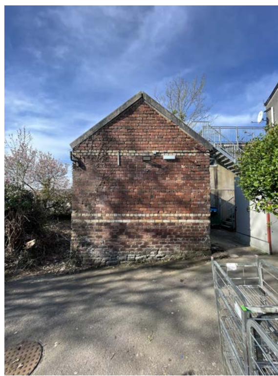
P1 Northeast elevation view
