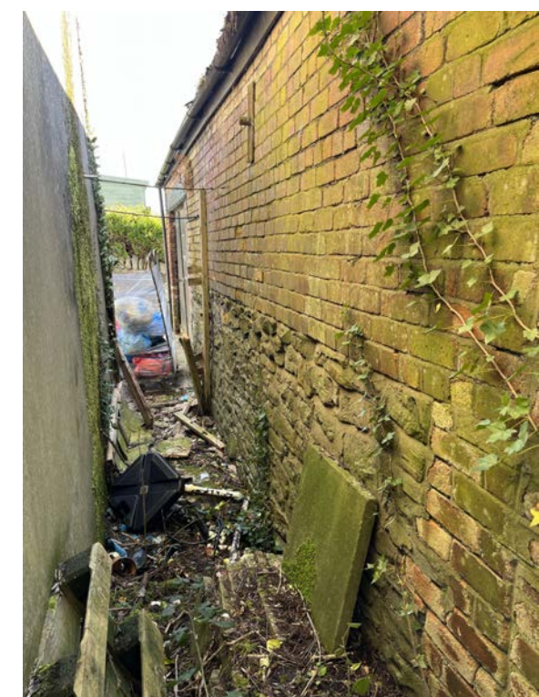
P14 Northwest elevation view showing the different wall materials and variable coarsing to the top of the stonework.
