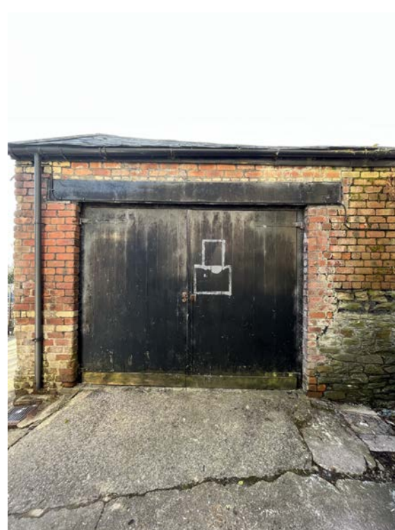
P15 Northwest elevation view of opening 4 (external) the double door entrance, lintel above and alterations to the reveals.
