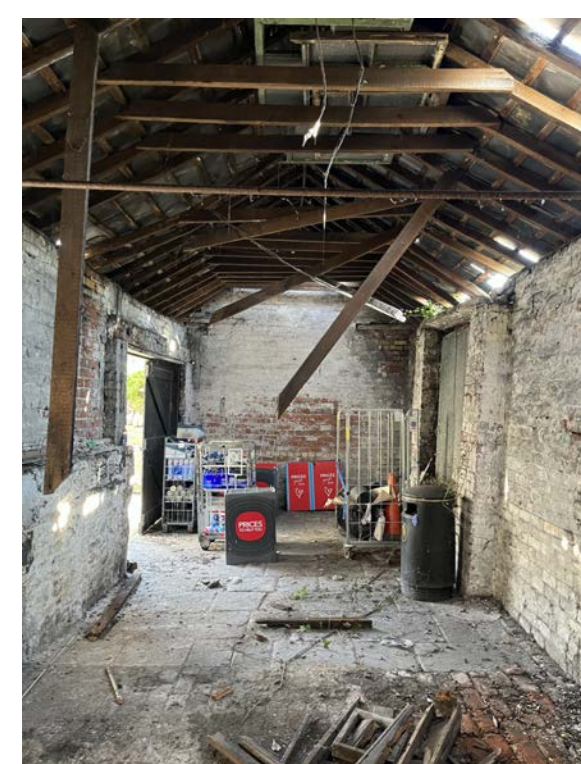
P17 Internal view facing east showing the space and roof trusses, floor surfacing division.
