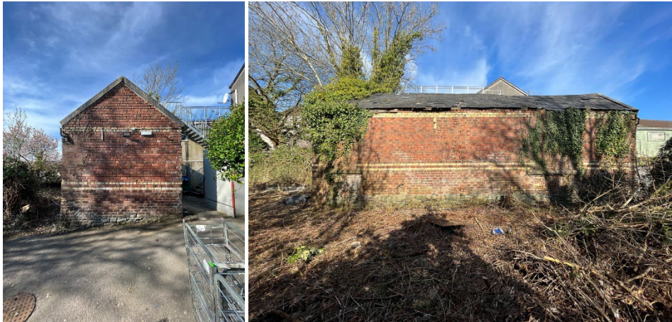
Photo 1: Northeast view of the gable end; Photo 2: Southeast view of the side elevation.
