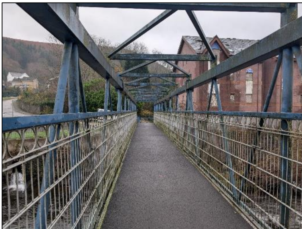
Photograph 4.2 River Taff footbridge
