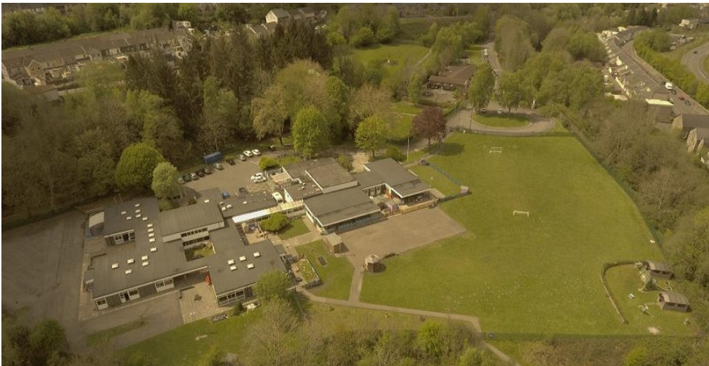
Figure 1-1 – Existing Site Aerial
