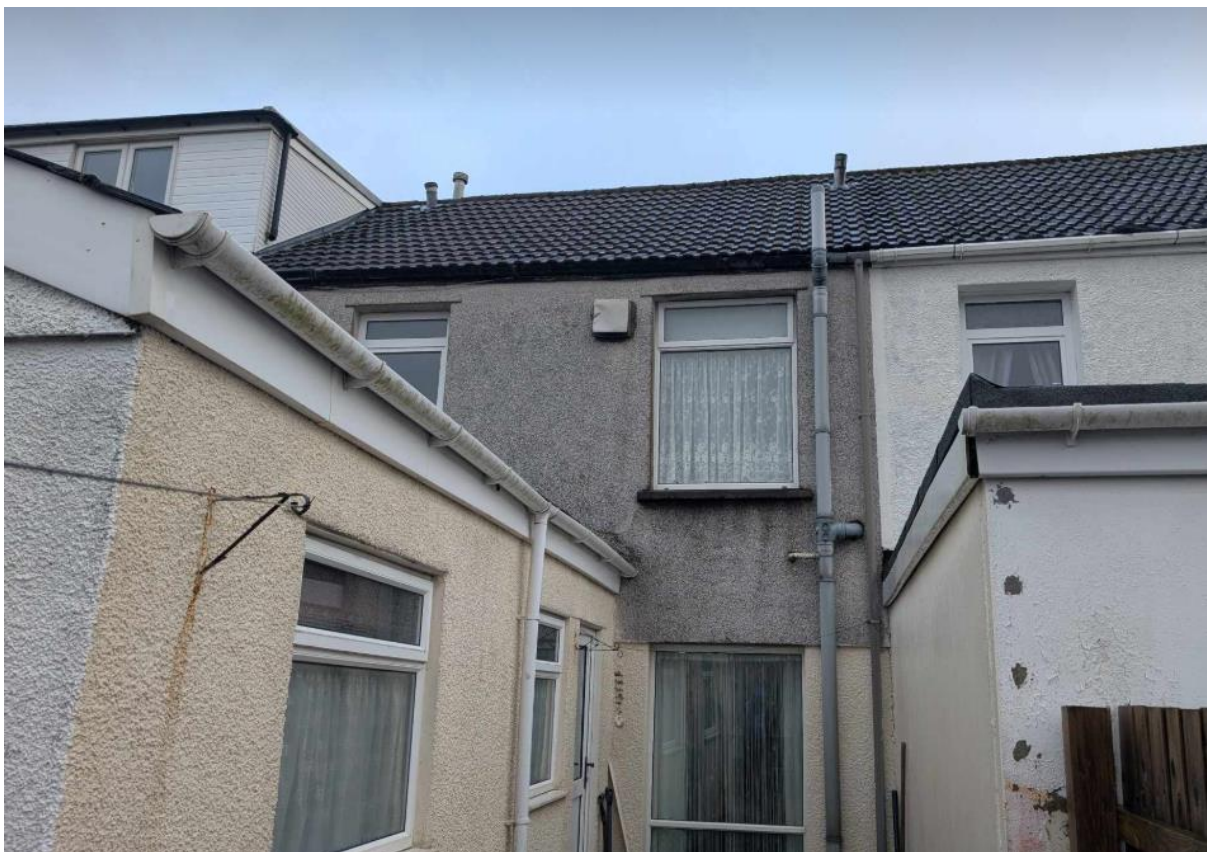
Plate 8- photograph of rear roof
