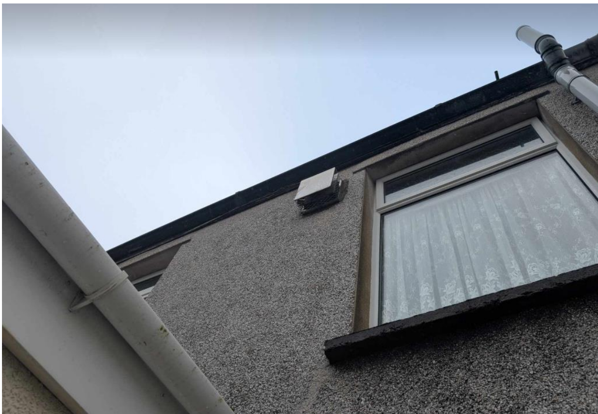
Plate 6- Photograph of gap beneath rear fascia board
