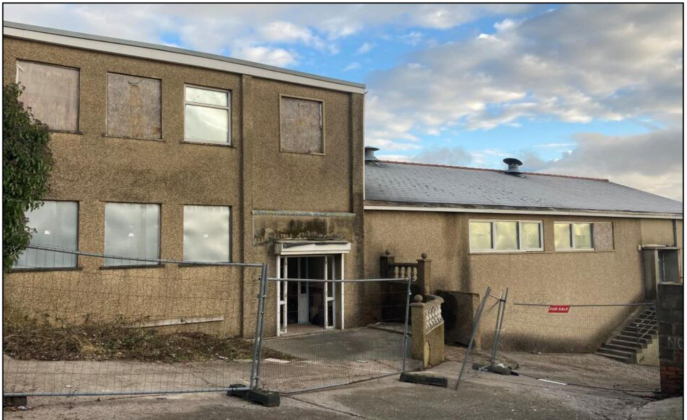
Photograph of existing main entrance area on front elevation
