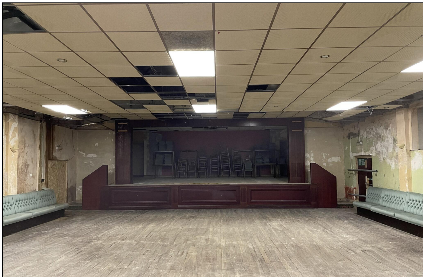
Internal photograph of the main hall area
