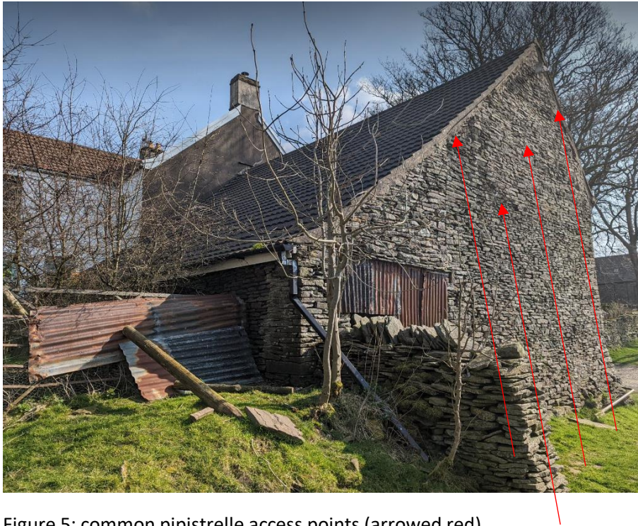
Figure 5: common pipistrelle access points (arrowed red)
