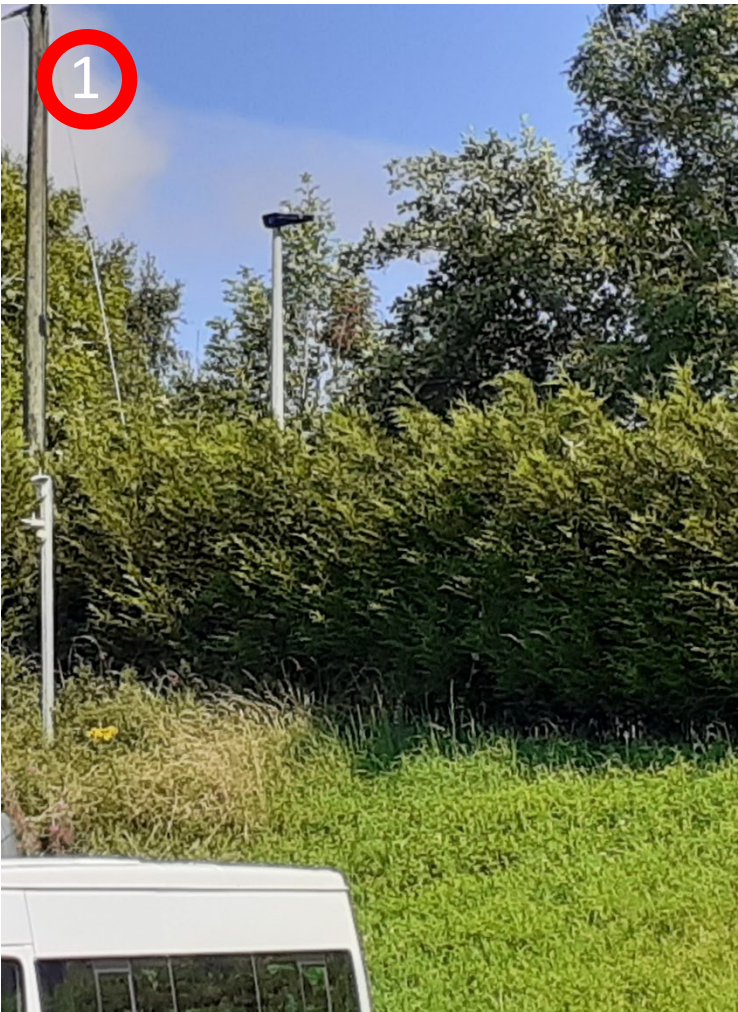
Existing lighting columns along pedestrian footpath
