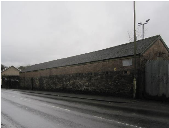
Plate 7: Western gable end, showing missing barge board
