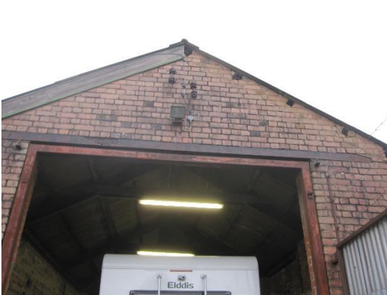
Plate 7: Western gable end, showing missing barge board
