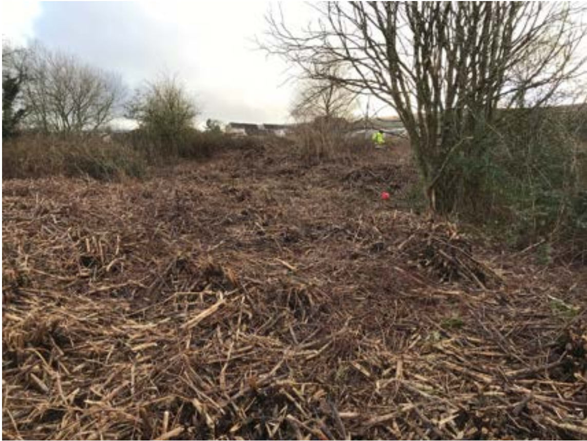
Top of JK1 – operator is working at the edge of the stand
