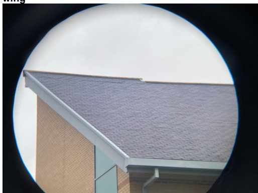
Plate 7: Gaps under ridge and roof riles on southern wing
