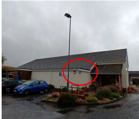
Plate 1- View Looking Towards The North Eastern Side Of The Building.
