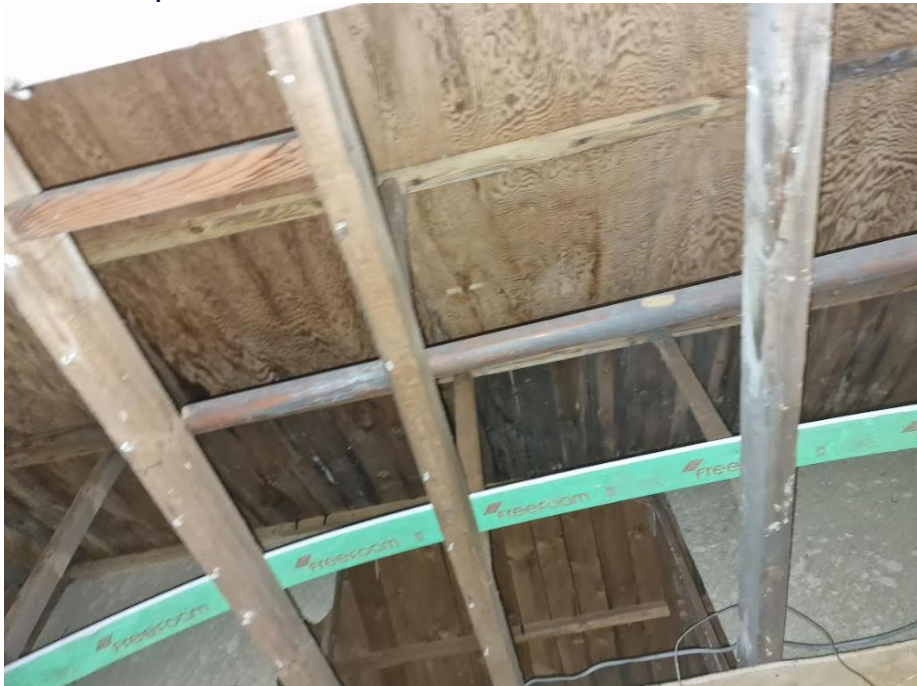
Plate 2- example of underside of cabin roof
