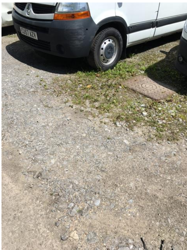
Photo 2 - Stone to dust permeable surface in part of lower yard
