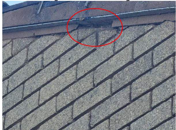
Photo 6: Missing mortar on western gable
