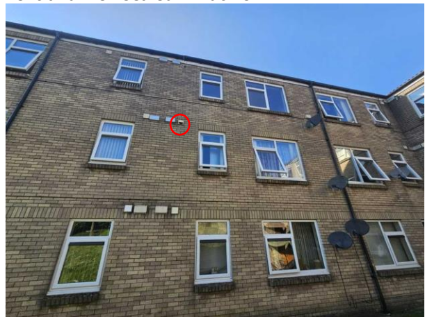
Photo 6: Missing mortar on western gable
