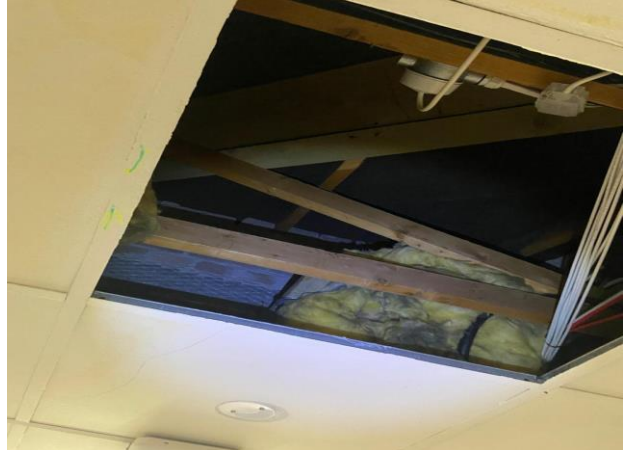
Photo 14: View into a section of the loft void above the suspended ceiling
