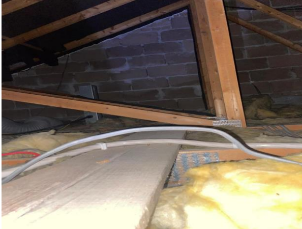
Photo 13: Internal loft space on eastern elevation, lined with bitumen felt
