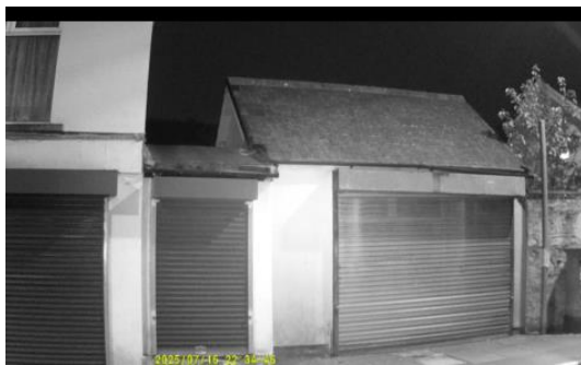
Plate A: Infrared Monitoring (NVA - Image quality)
