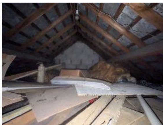
Interior roof space – Breathable membrane
