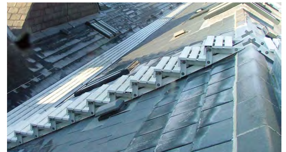
Image showing example of stepped walkway on pitched slate roof. The walkway will be finished in dark grey to match slating. Image taken from MSA Latchways.
