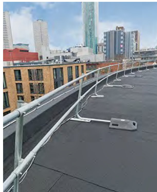
Indicative image of proposed guardrail system which will provide protection to edge of flat roof. Image by Alumasc.
