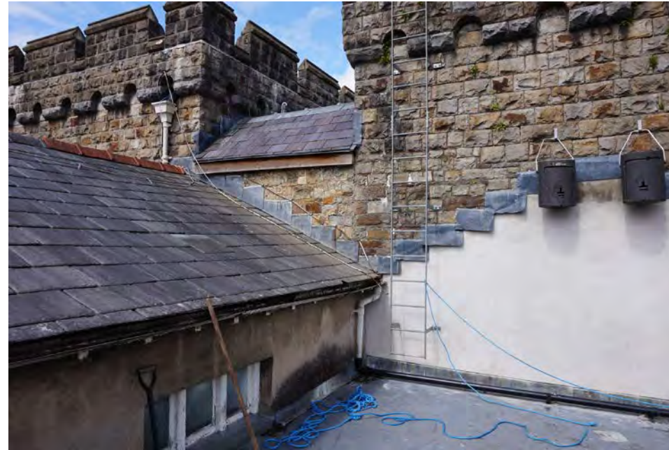
Image showing existing location of bat boxes on external wall of caretaker's house, new external bat boxes to be placed alongside existing. Location is only visible from roof.
