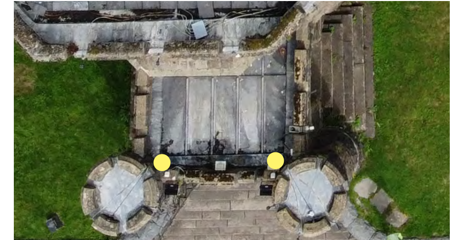
New RWPs 44 & 45 to direct water flow off towers thus preventing run off onto facade causing staining.
