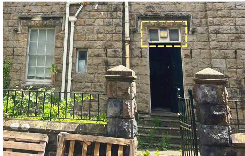
Example fo location where glass has historically been replaced with an infill and is to be reinstated.
