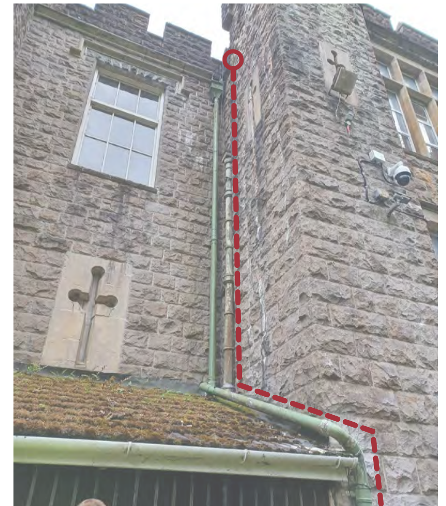
RWP 43: New chute, hopper and downpipe to manage water flow off flat roof area thus preventing water spilling over facade.
