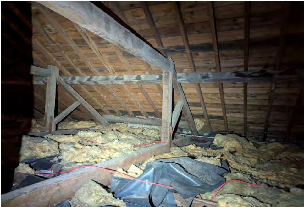
Image of roof space below R.7 where access walkway is proposed to enable safe access to roof space for maintenance and inspection.
