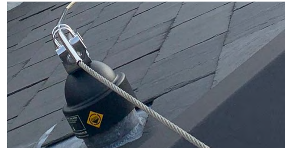
Image showing constant force post in slate roof. The post will be fixed through to the timber structure below.. Image taken from MSA Latchways.
