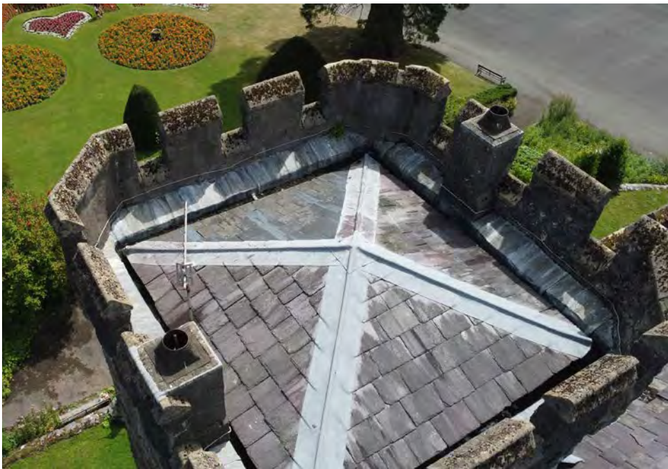
Roof pitch to be increased from rafters and slate roof above rebuilt.
