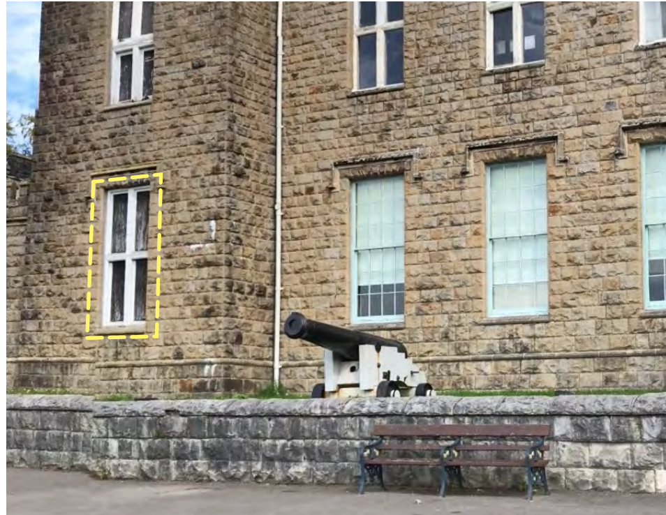
Existing boarded up window to caretaker's house (marked on image) is to be replaced with sash window to match adjacent ground floor windows.
