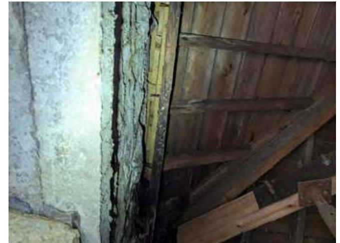
Underside of roof covering in void R.1.9 (the pitch of this roof is proposed to be altered to allow for more effective water run-off).
