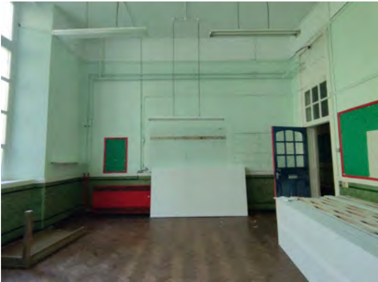
Typical example of a classroom within the former school.
