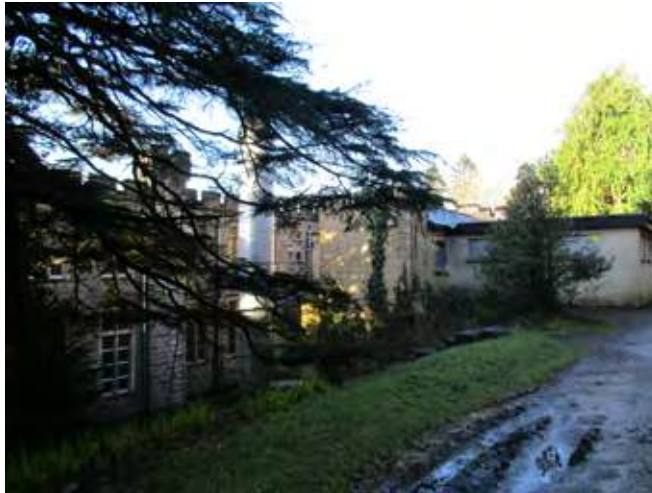
Rear elevation (partial), note the first floor extension to the rear of the School
