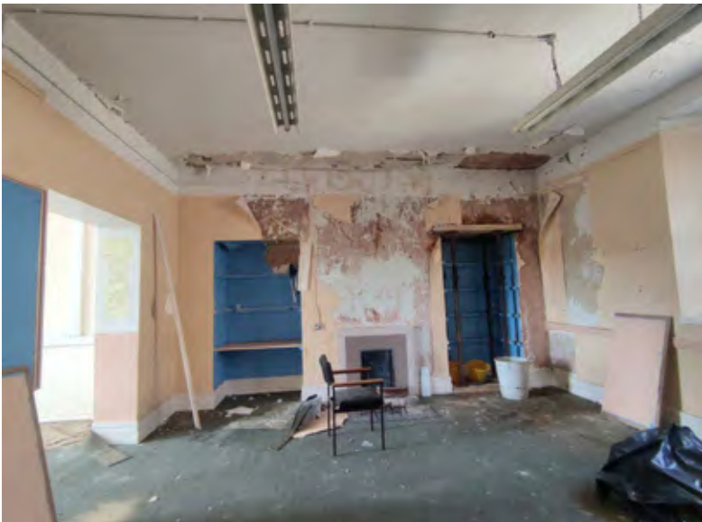
Looking west within room 1.55A at first floor level (where structural interventions are proposed to the ceiling).
