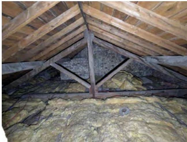
Interior of roof void R.1.20 (south range)
