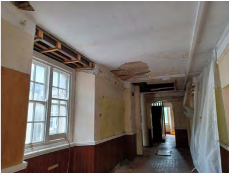
Looking east within corridor 1.31C., where structural works are proposed to the ceiling.
