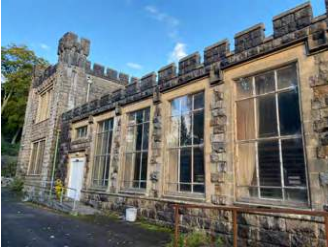
The west elevation of the Castle.
