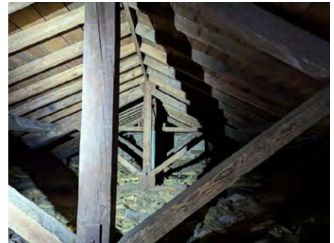
Interior of roof void R.1.15 (south range)
