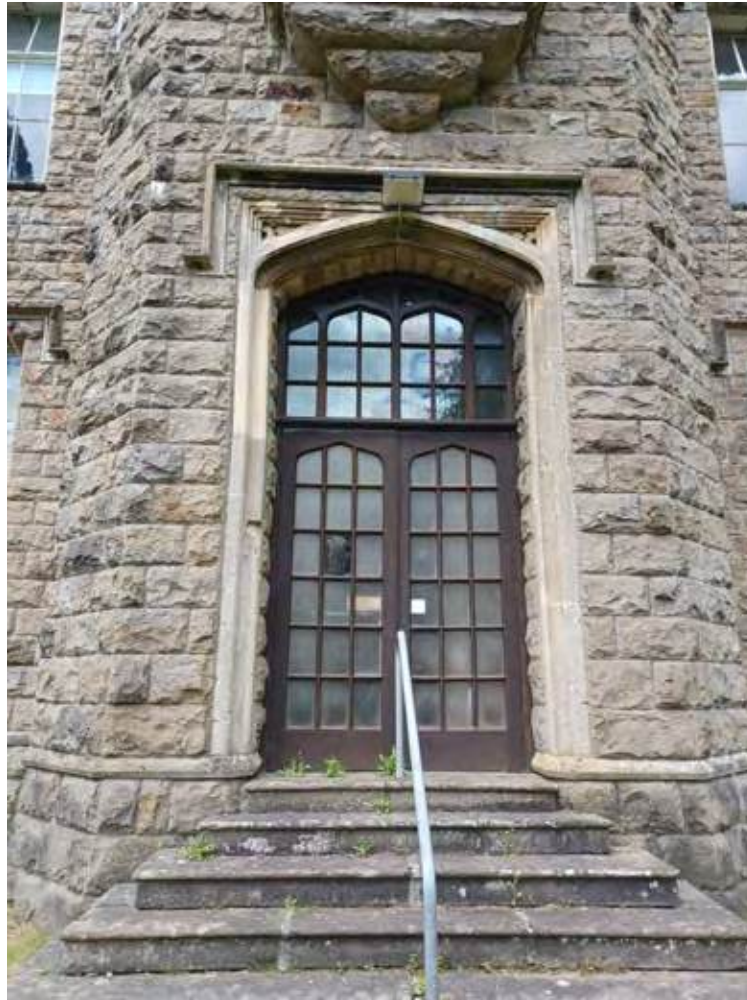
The door to the south-eastern facade, which is a 20th-century replacement proposed to be removed as part of the scope of works.
