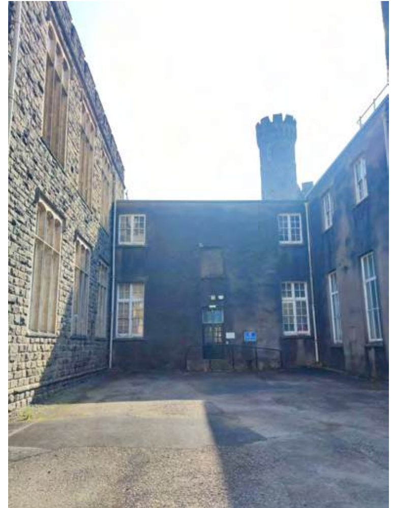
Looking east within the main courtyard towards the set of historic double doors proposed for replacement.
