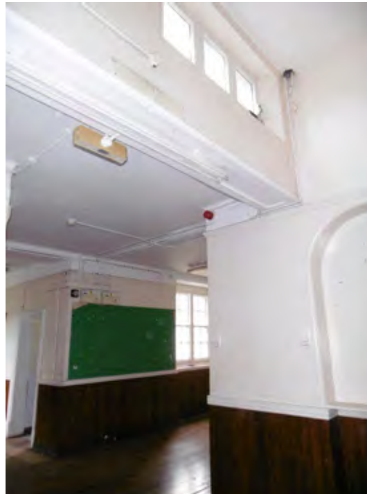
Looking south-west within corridor 1.31E at first floor level. The high level window is proposed to be altered as part of the proposed works.
