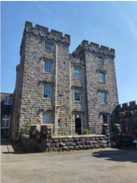
The west elevation of the Caretaker's House, from the central courtyard.
