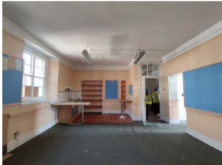
Looking east within room 1.55A.
