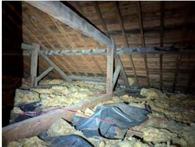
Roof R.1.7 (south-east range)
