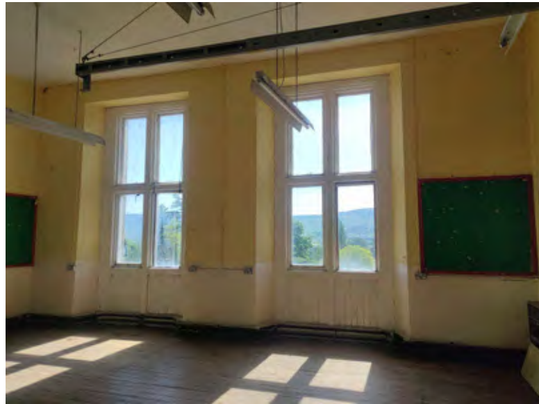
Room 1.41 - the proposed location for a new loft hatch.
