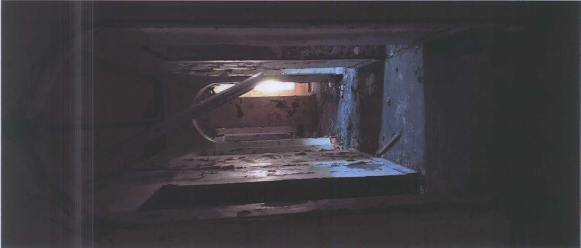
View north along corridor
