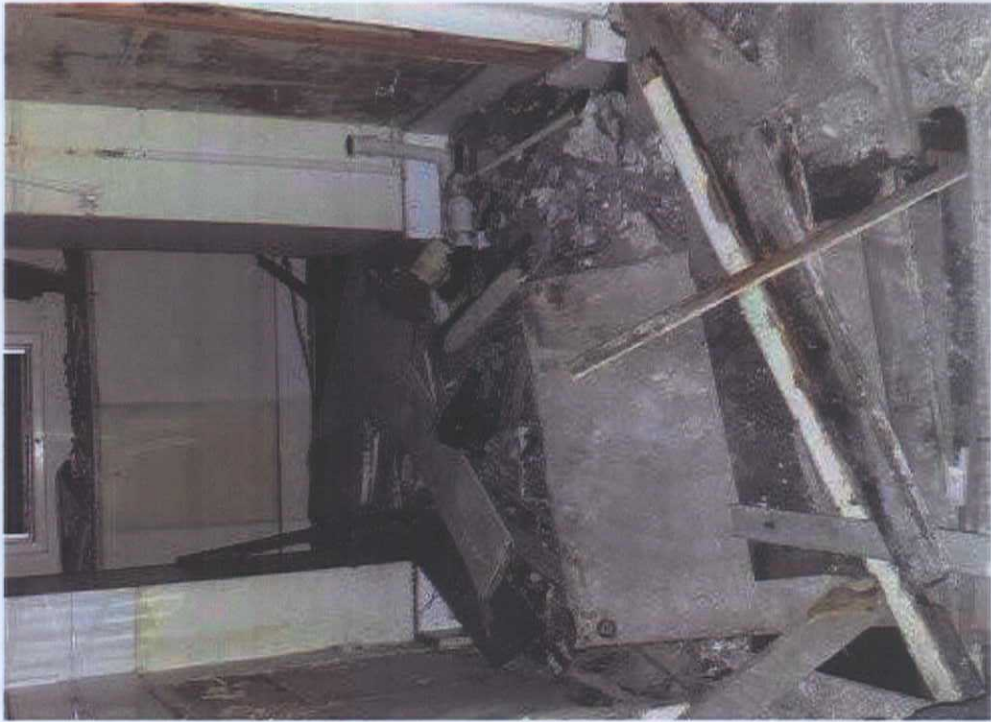
Collapsed drainage inspection chamber in floor
