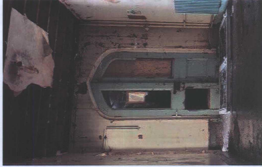
West Wall & Ceiling
