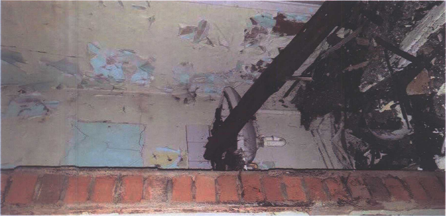
Looking south into WC
