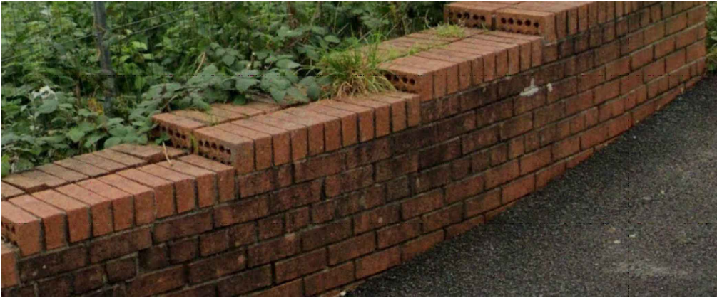
Face brick matching existing boundary wall
