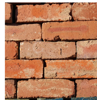
Brick Quins and Soldiers Reclaimed orange bricks
