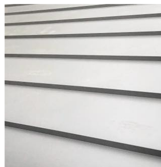
9. Snaplock standing seam roof, Coated Aluminium - Zinc Patina
