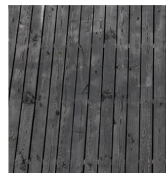
6. Shou Sugi Ban Charred timber cladding (vertical)
