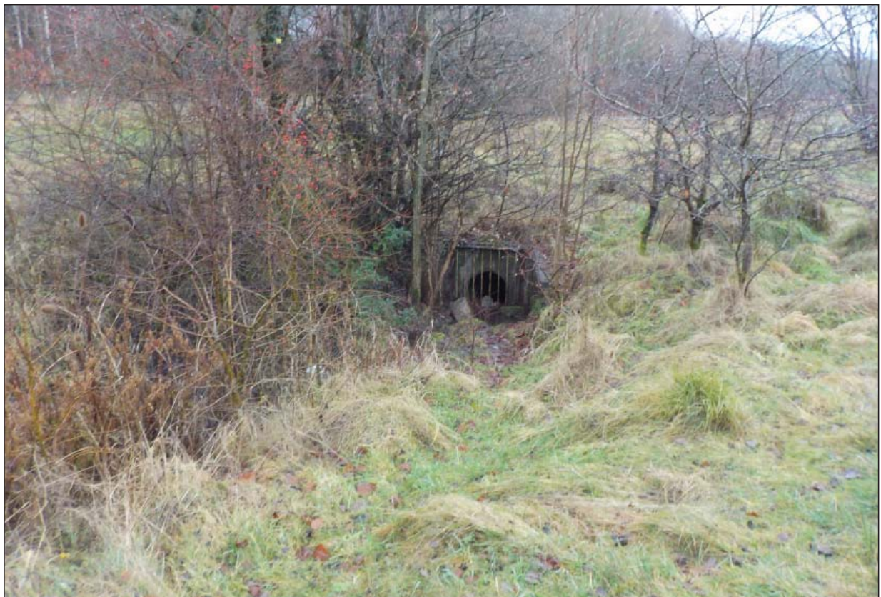
Plate 2 - Culverted watercourse in the north of site, looking southeast
