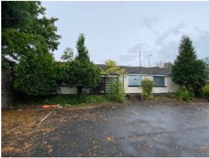
Chalets and flower beds along north west boundary viewing north west
