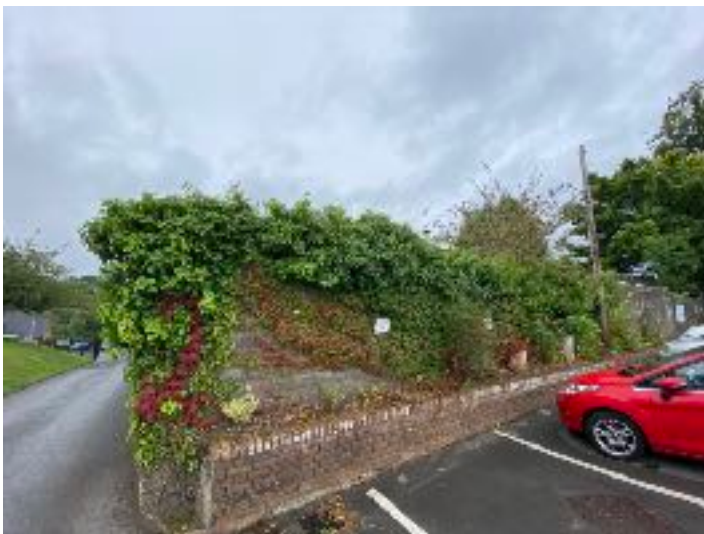
North western boundary wall viewing east from football ground car park
