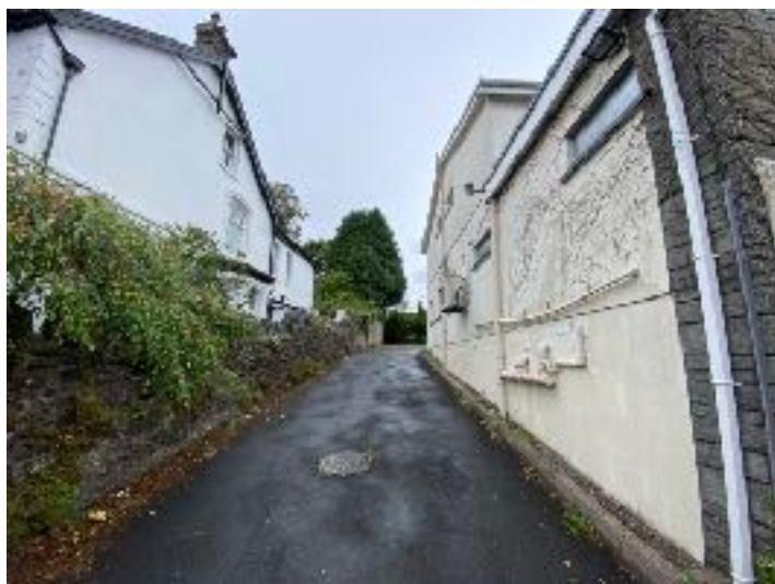
South western elevation of hotel viewing west
