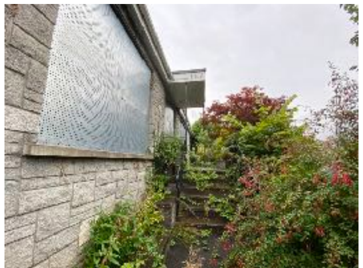
Slope up to hotel entrance and overgrown ornamental shrubs
