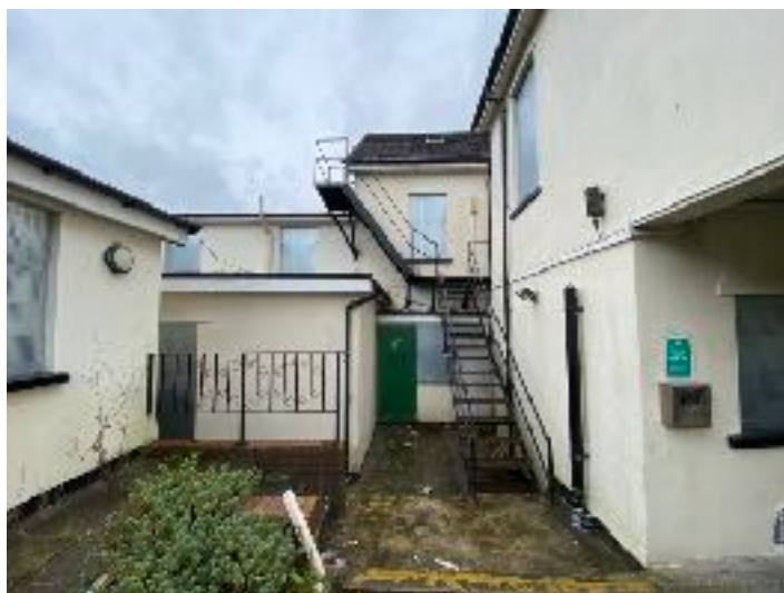
North eastern extensions to hotel viewing east
