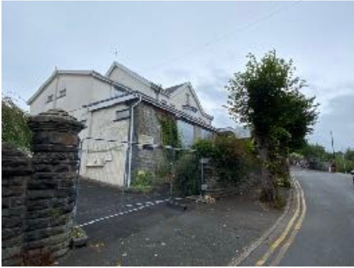
South eastern elevation of hotel frontage viewing north
