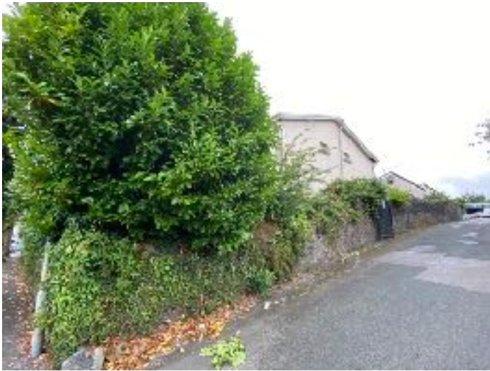
North eastern elevation of hotel viewing west
