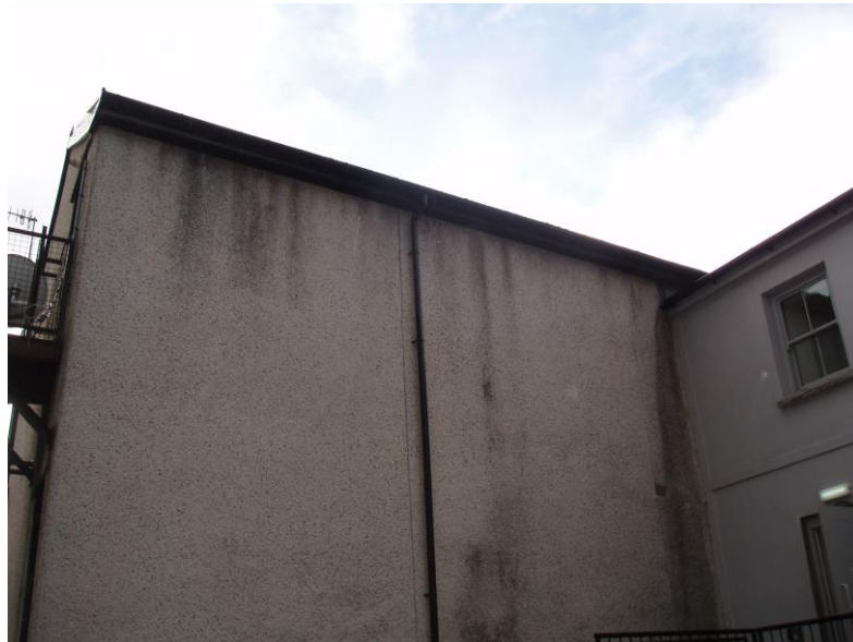
North facing elevation, new soffit, tightly sealed
