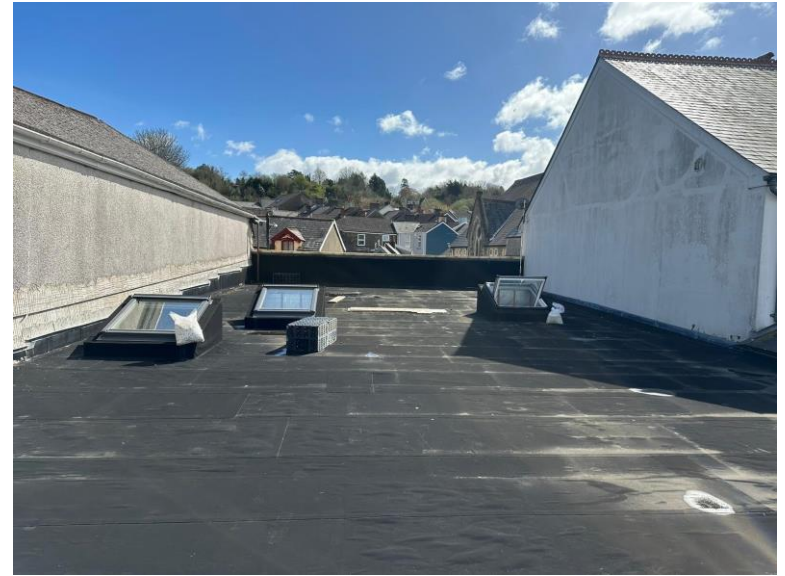
Existing flat roof
