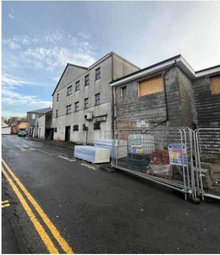
Rear elevation-facing West
