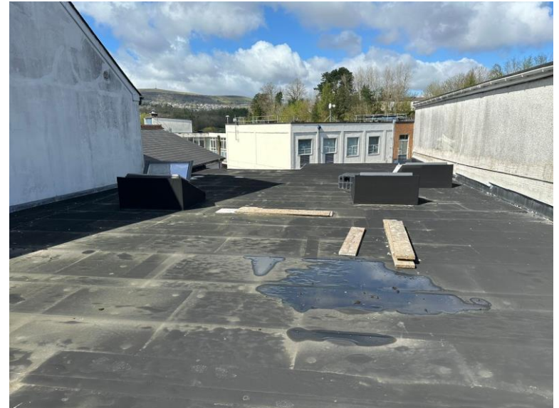
Existing flat roof
