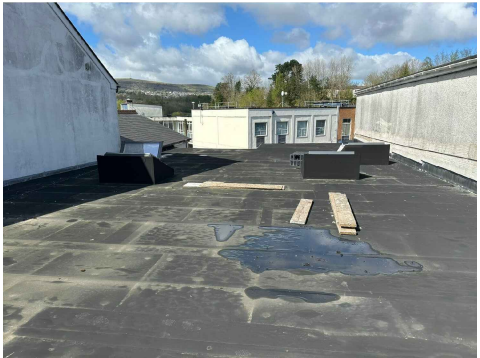
2 IMAGE OF EXISTING ROOF
