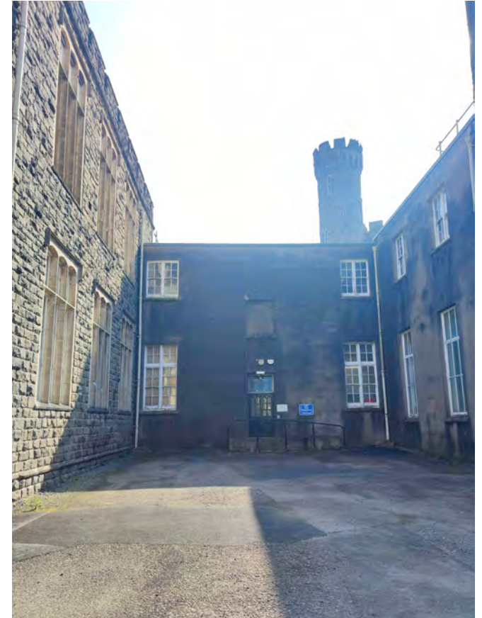
Looking east within the main courtyard
