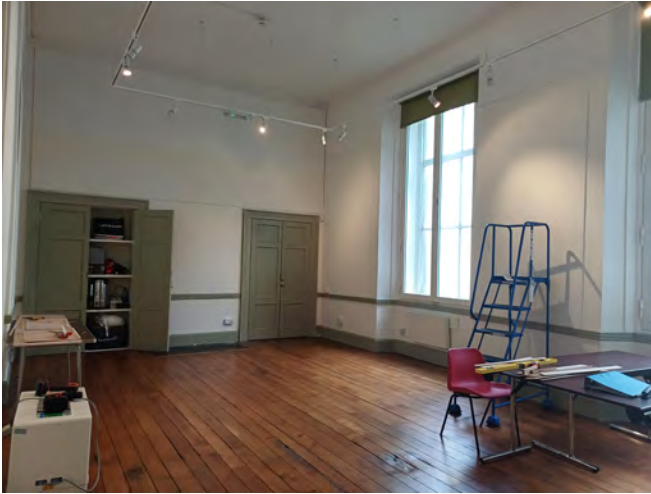
The Play Room Gallery, which was converted to serve as a gallery during the 1990s. The finish is plain compared to the other ground-floor rooms, but the space retains historic timber flooring, skirting, cornicing, doors and joinery.
