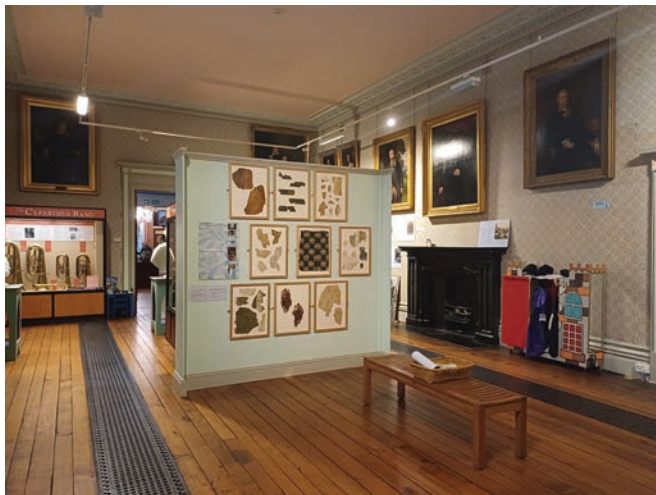
0.20 - Dining Room Track to be replaced like-for-like
