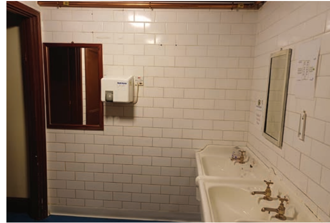
Heritage sinks and fittings to be retained. Tiled wall to be refreshed
