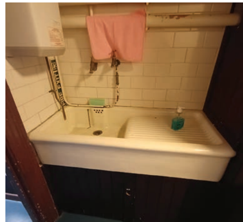
Belfast sink to be retained
