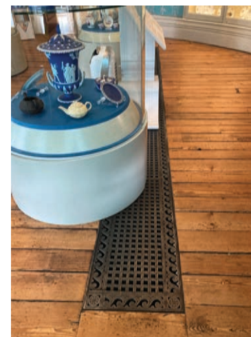
Cabling to be run in floor grilles.
