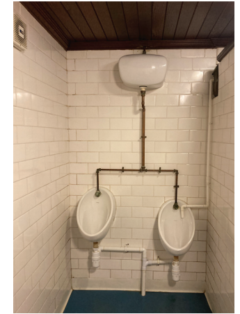
Historic urinal fittings to be retained
