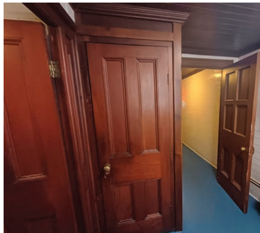
Heritage doors and other woodwork to be retained and restored with wax
