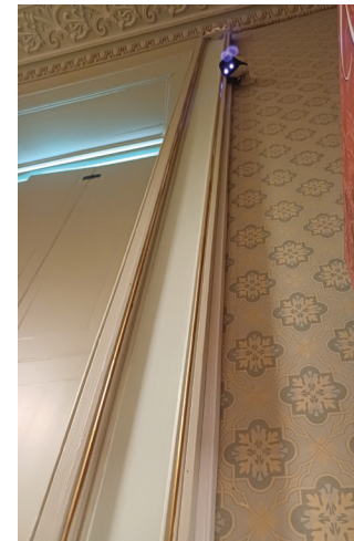
Examples of trunking which is installed alongside architraves resulting in a discrete finish.
