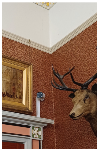
Example of locations where trunking is to be wall mounted. Trunking will be covered with wallpaper or painted in same colour as wall
