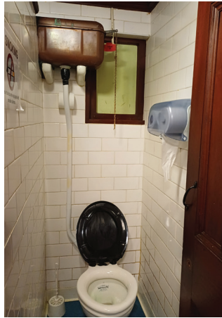
WC with high-level aluminium cistern to be retained
