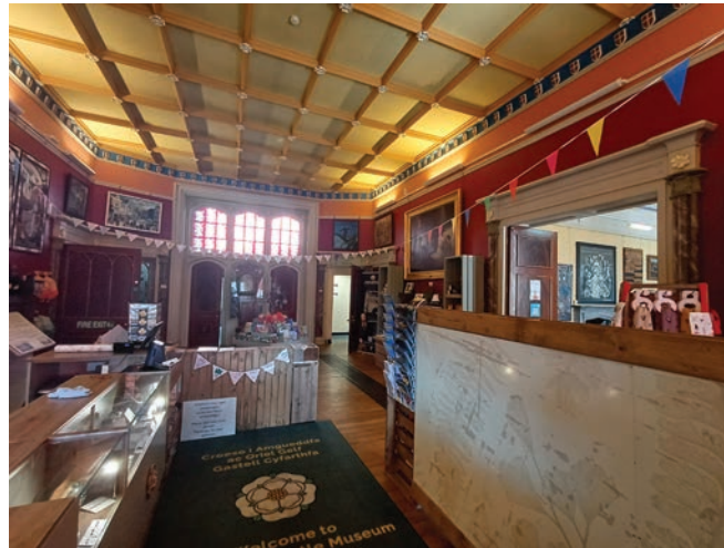
0.46 - Entrance Hall Tracks running alongside picture rails to be replaced.
