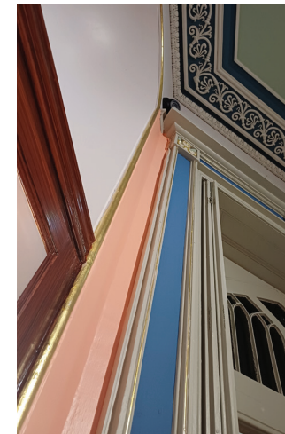
Examples of trunking which is installed alongside architraves resulting in a discrete finish.
