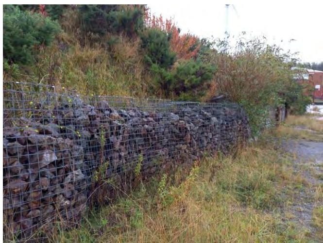
Gabion wall within north west of site.
