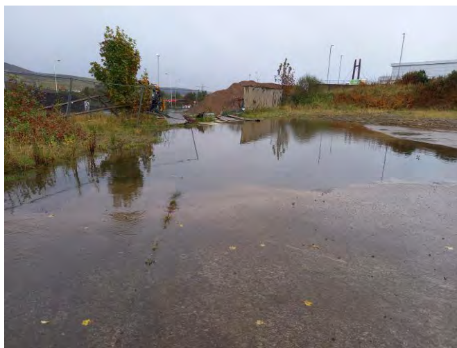
Flooded area in centre of site.
