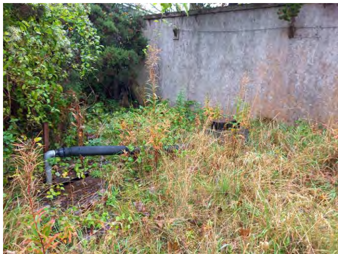
Drainage in east corner of site.
