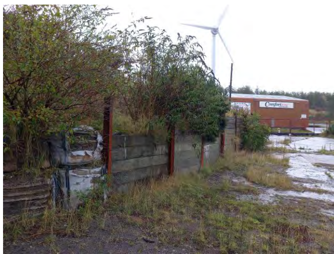
Retaining wall within north west of site.
