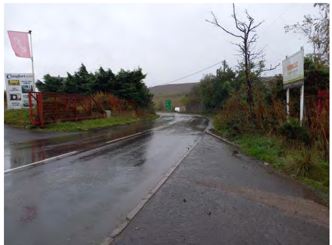
View from north of site looking east.
