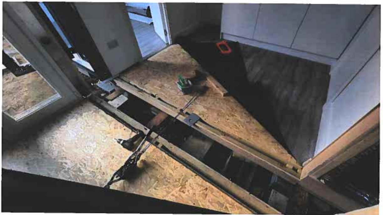
Note ratchet pulley to pull halves together and line of bolts in vertical plane awaiting tightening
