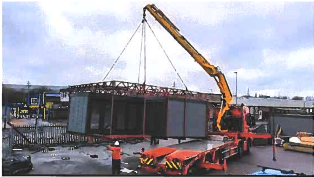
Same model caravan being lifted whole onto lorry for transportation
