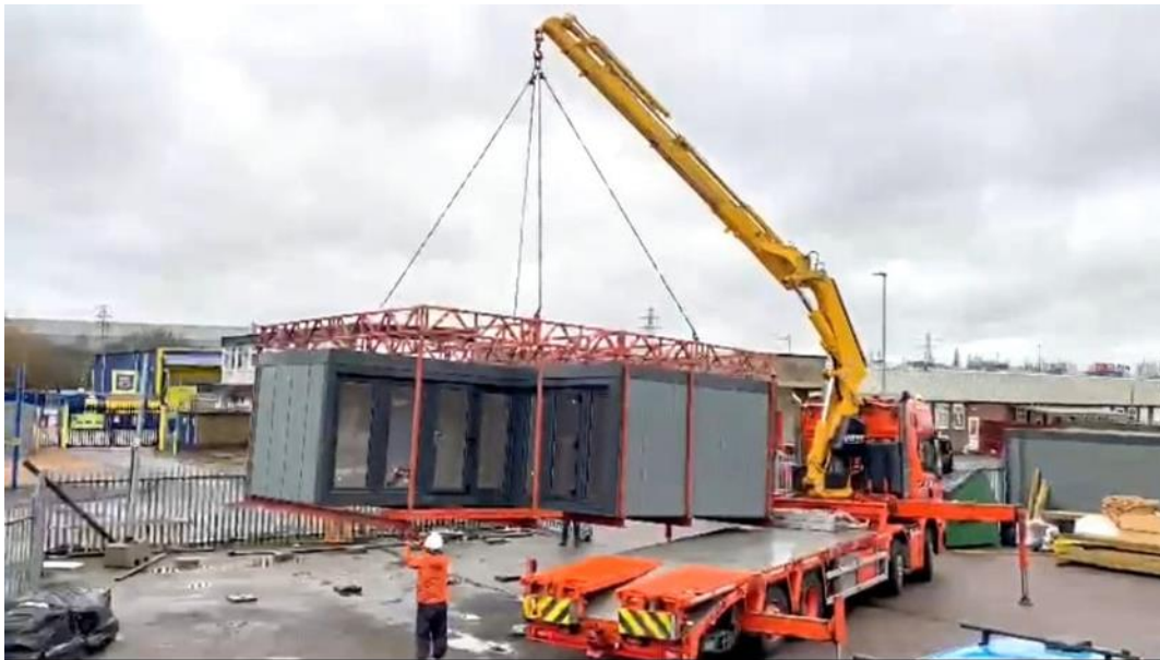
Photograph of lifting in operation
