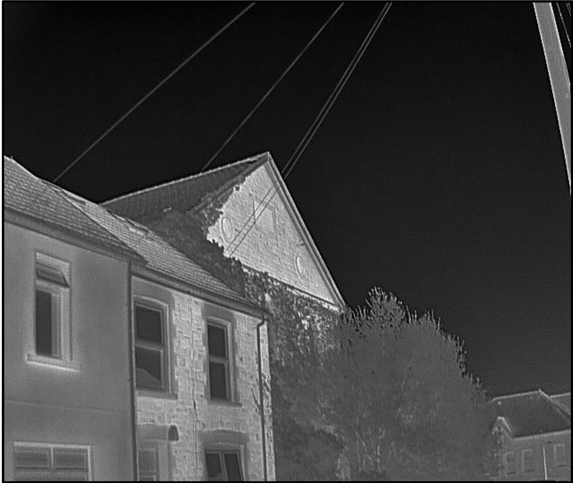
External thermal image taken at the darkest point of the survey (Collins 2023, Section 7.2.10).
