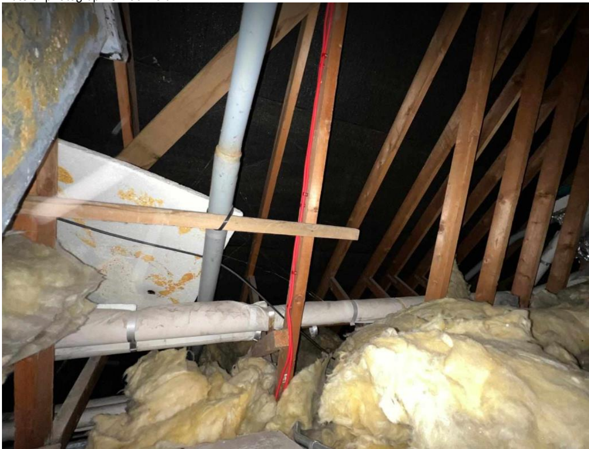
Plate 6- photograph of roof void
