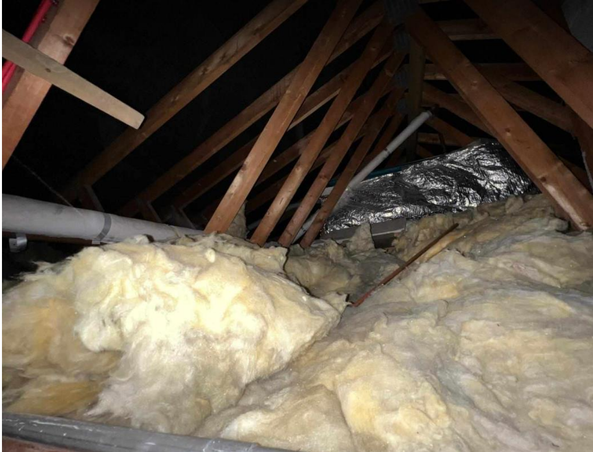
Plate 7- photograph of roof void
