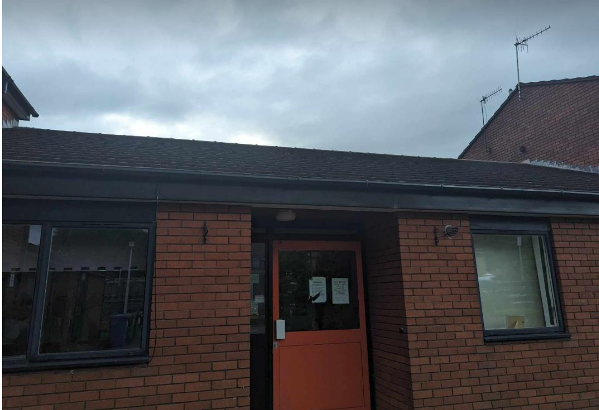
Plate 5- photograph of single storey building linking two two storey buildings
