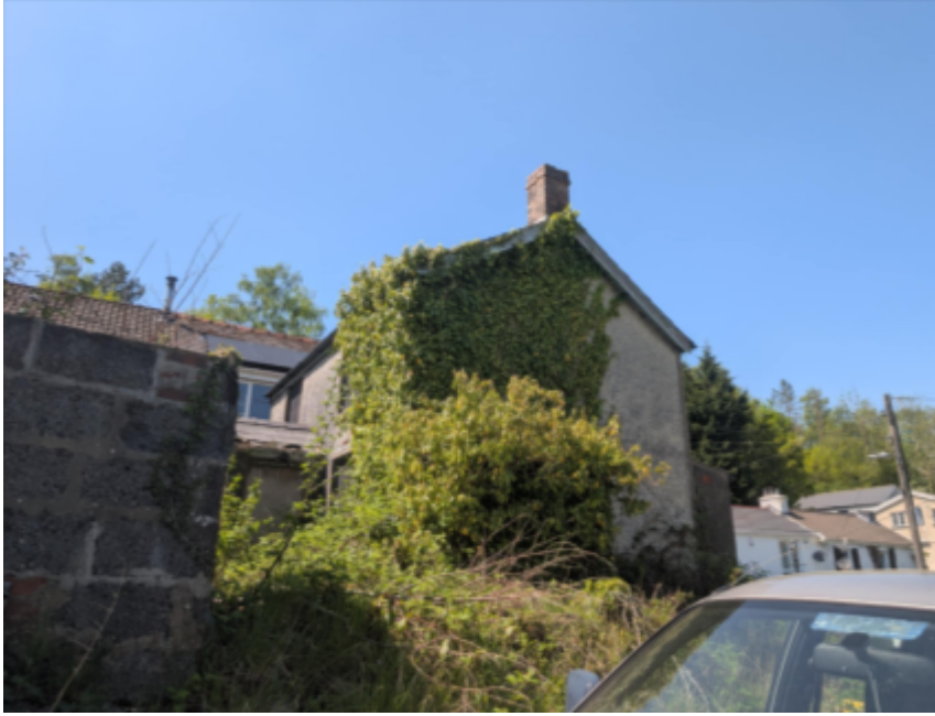
plate 7- southern elevation of house
