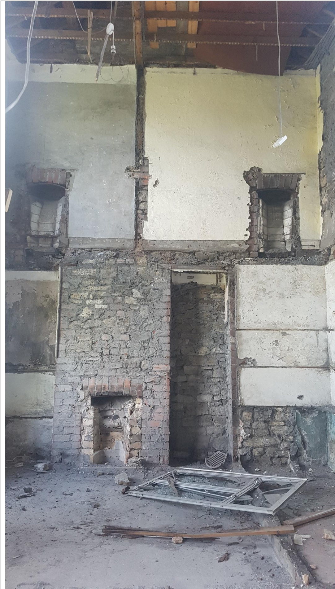
Photo 8. Ground and former first floor interior
