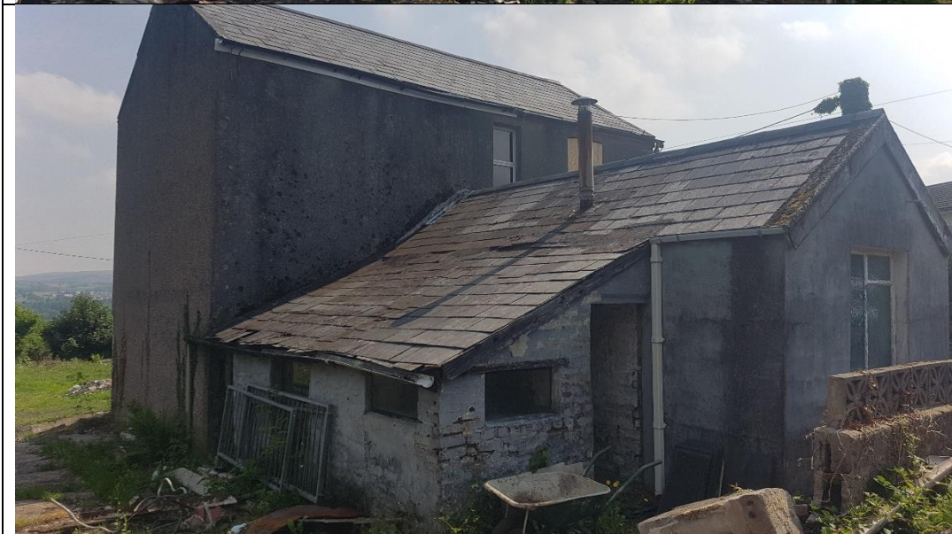
Photo 2. Side and rear elevations showing extension (west and south). Open doorway to outhouse only. No access to house interior
