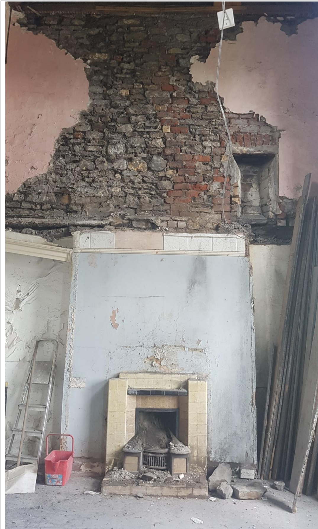
Photo 7. Ground and former first floor interior
