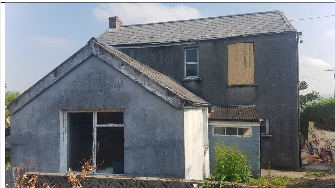
Photo 3. Rear elevations (south)
