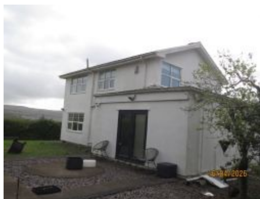
Building A – Northern elevation
