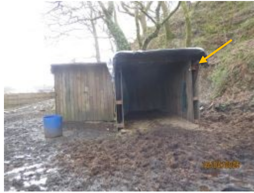
Building B – Western elevation – PRF – Potential night roost. Arrow shows location of inactive nest.
