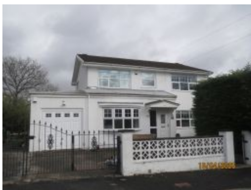
Building A – Southern elevation
