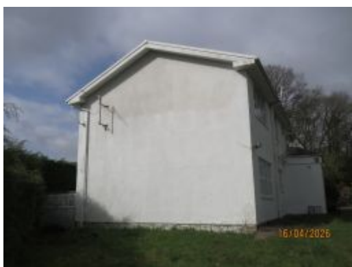
Building A – Eastern elevation
