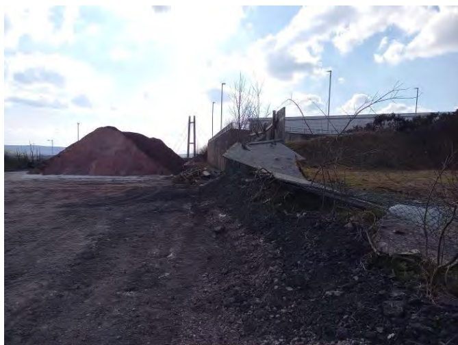
View from east of site looking south west.
