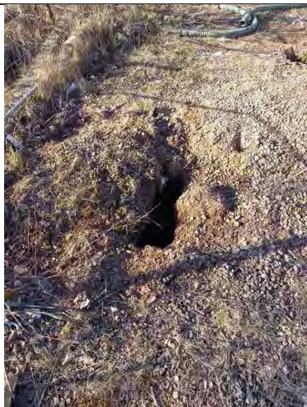
Manhole near BH03A
