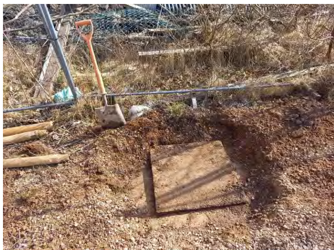
Manhole near BH03A
