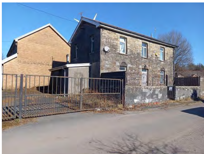
House in eastern section of site.
