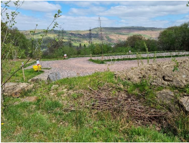
Figure 15 – View south across new car park area.
