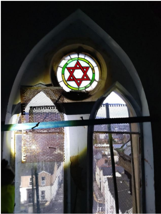
Figure 26 - Gaps in window on second floor.
