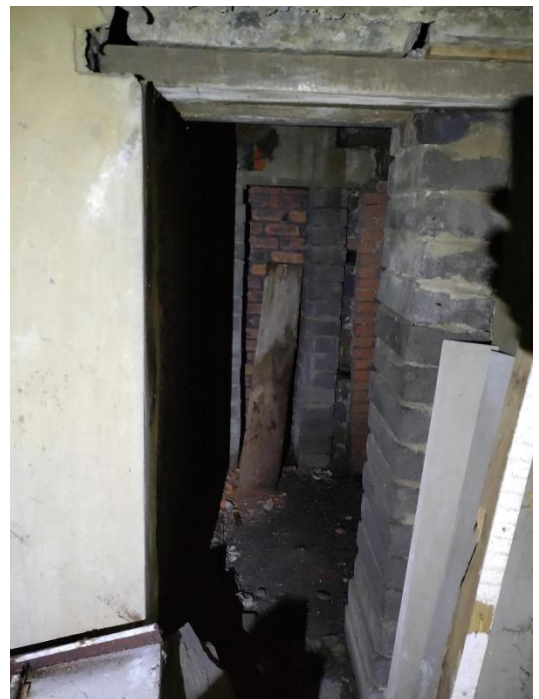
Figure 33 - Gaps in brickwork in northern basement.
