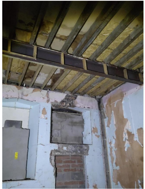
Figure 15 - Exposed brickwork on ground floor.
