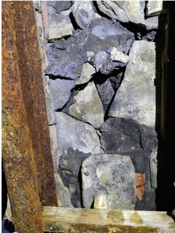
Figure 34 - Gaps in brickwork in northern basement.
