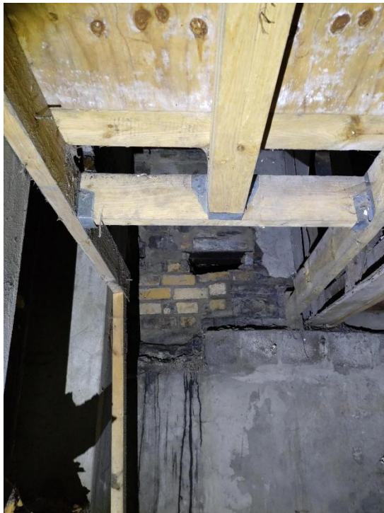
Figure 32 - Gaps in brickwork in northern basement.
