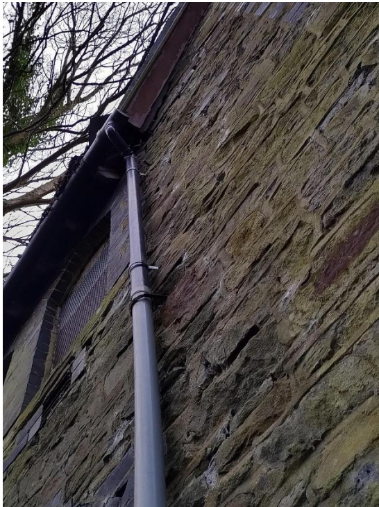
Figure 38 - Gap between wooden soffit and wall on northern aspect of the building.
