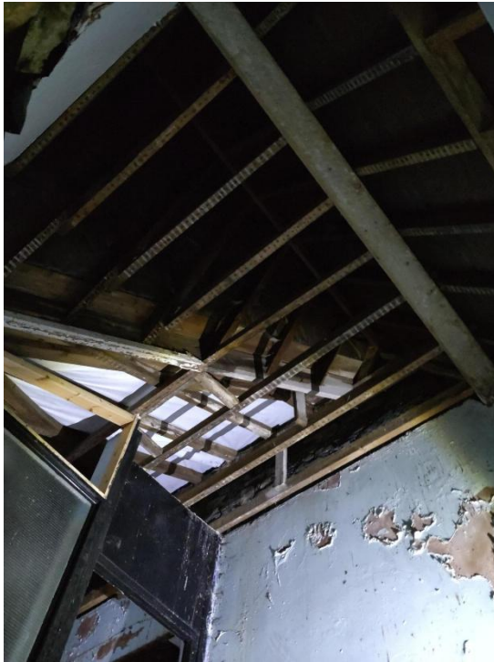
Figure 22 - Wooden beams on second floor.
