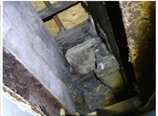
Figure 214 - Gaps in stonework on first floor.
