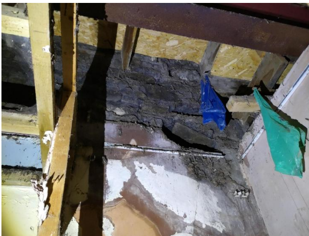
Figure 20 - Gaps in brickwork on first floor.
