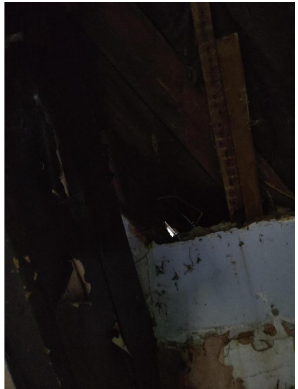
Figure 31 - Gaps in roofing felt on second floor.
