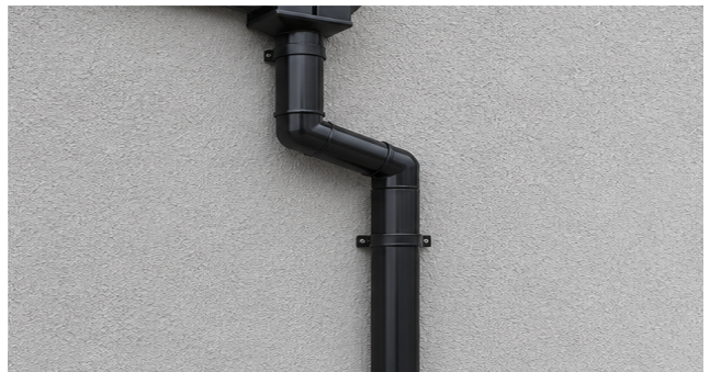
06 Downpipes Black uPVC
