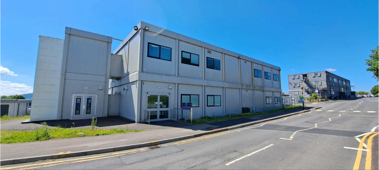
Unit 3 view from north-east
