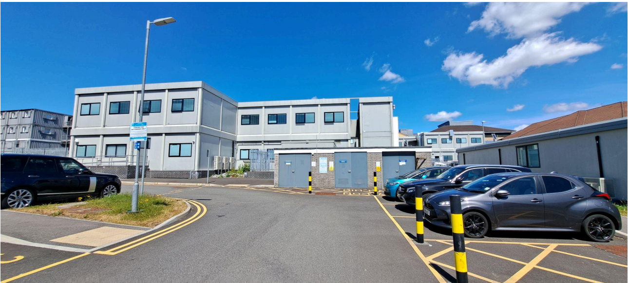
Unit 3 view from south
