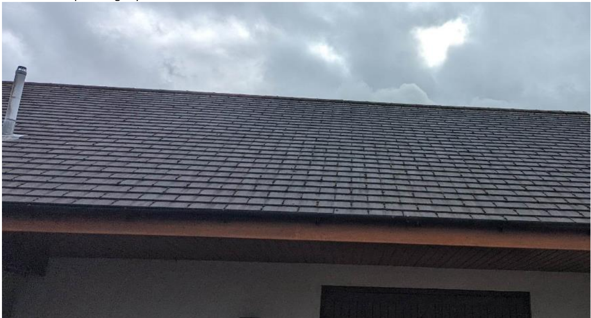
Plate 8- example of tightly fitted roof
