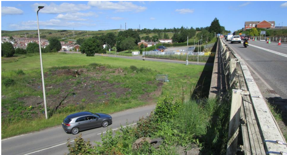
View east along A465(T) showing Cheltenham Avenue (foreground) the MMA yard (middle) and housing to south of road at the higher level (July 2021)
