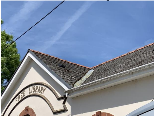
Photo 5: Roof tiles and lead flashing
