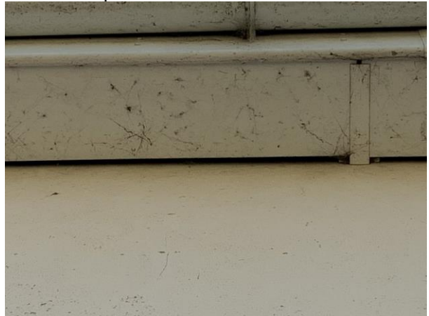
Photo 6: Gap behind uPVC soffit
