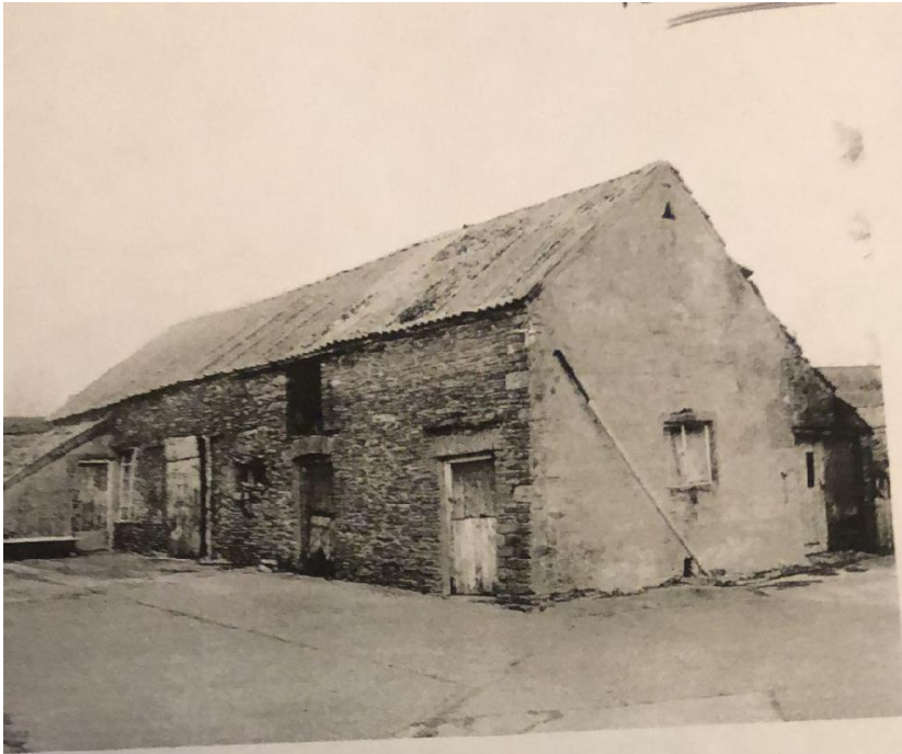
Photo 12: Building J taken from south – to be converted to Unit 5.
