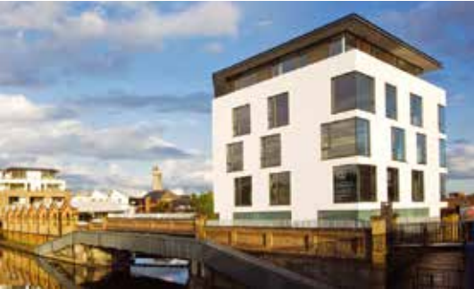
Westbourne Grove Canal Building, London
